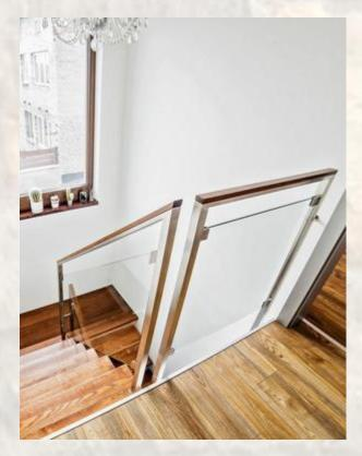
Railing stainless steel railing, handrail covered with wood
